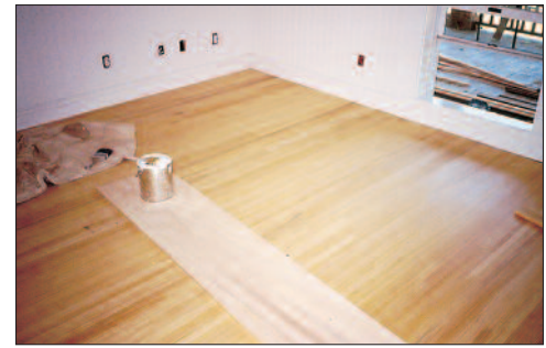
During finishing, avoid unnecessary contact with the floor by using a fabric runner. Stains and waxes cannot penetrate perspiration, hand and knee imprints.
